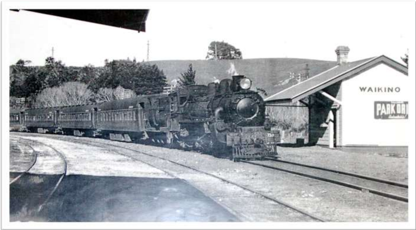
Waikino Rail Station
