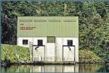
LDC Lower Mangapapa Power Station, 1988. On the left-hand side of the image there can be seen a tall concrete wall. The bulk of the main structure is positioned above the existing structure in the foreground.
