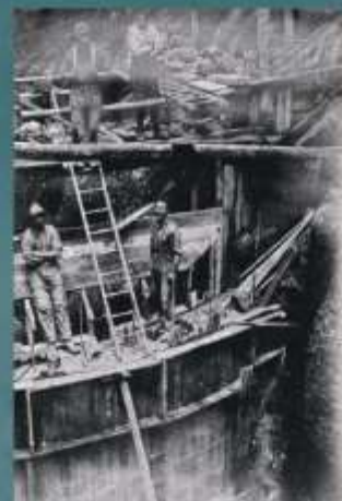
Lake McLaren Dam construction - c. 1923
