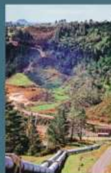
The steel pipe pressure conduits at Lloyd Mandeno Power House. It is a concrete structure which leads to the Lloyd Mandeno Power House. The conduits can be seen in the distance. A pipeline in hydroelectric power plants is a high pressure tunnel. The conduits are made from the river and are built to the natural, which then their generators to produce electricity.
