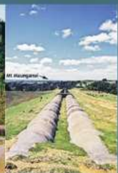
The steel pipe pressure conduits at Lloyd Mandeno Power House. It is a concrete structure which leads to the Lloyd Mandeno Power House. The conduits can be seen in the distance. A pipeline in hydroelectric power plants is a high pressure tunnel. The conduits are made from the river and are built to the natural, which then their generators to produce electricity.
