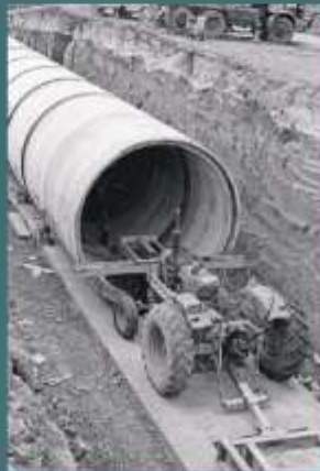
Rolling of concrete pipe on road at period of construction, 1962
