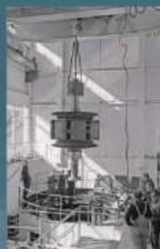
Installing a generator in the Lloyd Mandeno Power House, Aug 1976.
