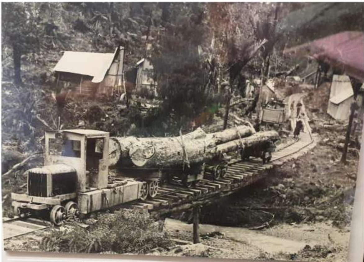
A petrol driven locomotive using a truck engine working at the Mata bush near Waipu, 1936. The Contractor was Bert Collins for Kauri Timber Company.
