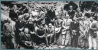
A group photo of the construction of the Omana Falls power station, 1911, with H.W. Climie and sons.
