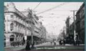
Laying of Queen Street from the Carlton Street tramway, Auckland. A tram car is visible in the distance. Lloyd Mandeno was one of the engineers of the city's first AC tram system.
