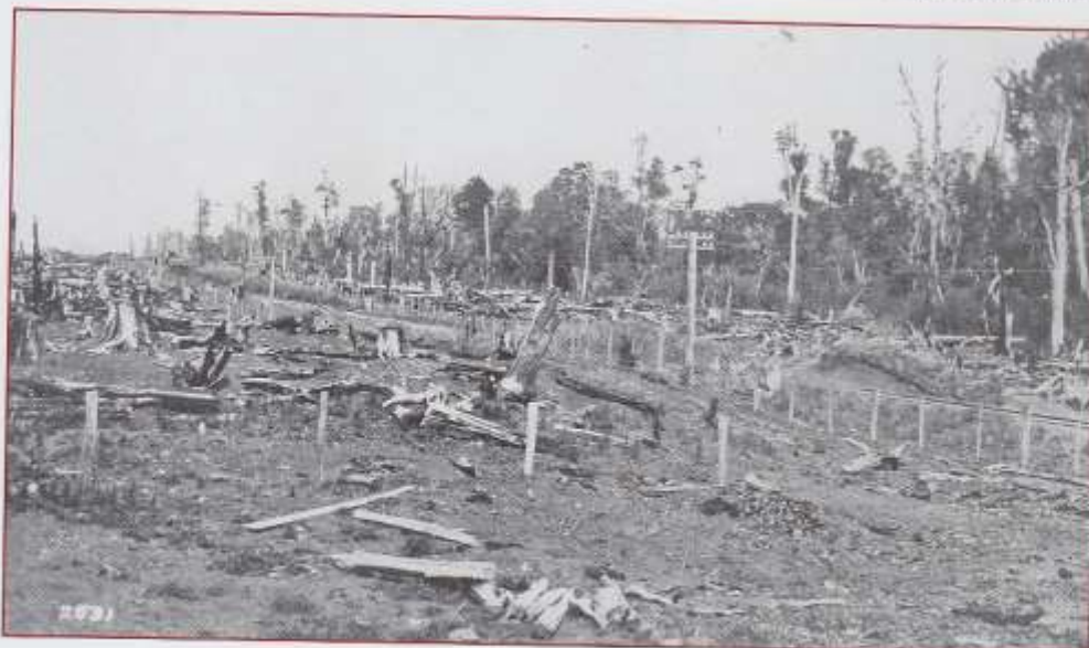
Anderson's charcoal pit, the origin of the 1926 fire, alongside the NIMT 0.8 km north of Pōkākā. Photograph: Archives New Zealand, R2421979, AAQA, W3347, 6504, Box 7
