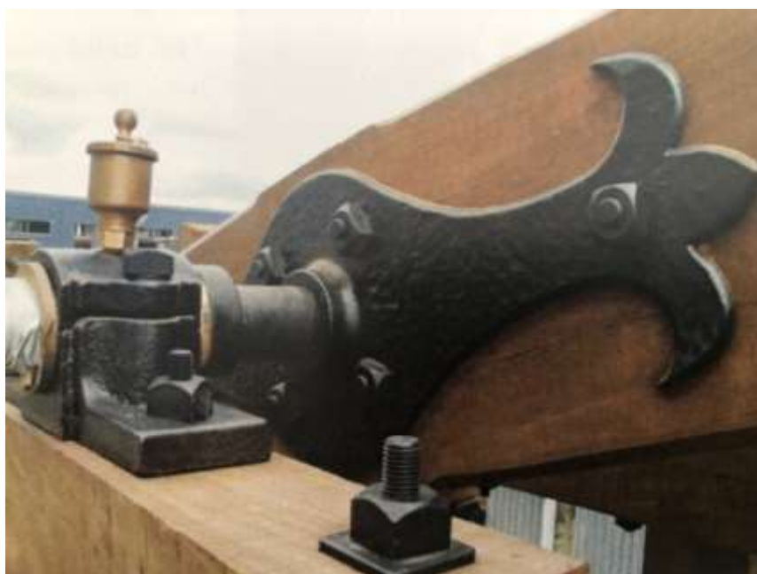
Fig 5 shows the beam pivot with its hand crafted plate and shaft work. The bearings had been repurposed as well.
