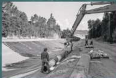
Working on the dam, 1978.
