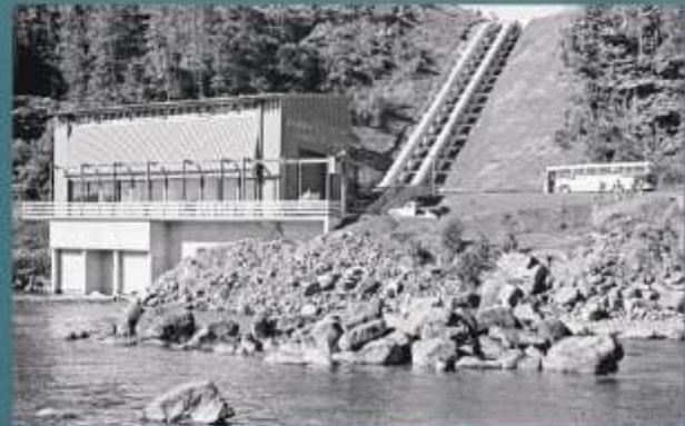
Side view of the Ruahihi Power Station, 1981.
