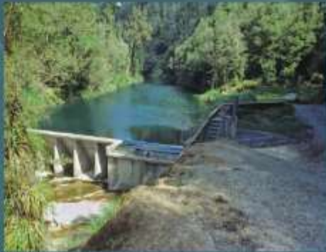
An intake and penstock structure of Ōmanawa Falls, where the main flow of the Ōmanawa River is diverted to feed the other turbine (Taylor & Francis, 1987)
