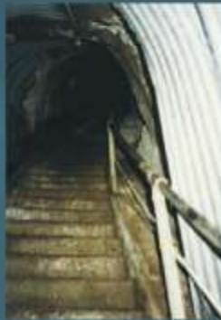
The access tunnel to the Ōmanawa Power Station
