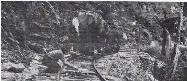
Figure 9: Preparing to lower logs down the incline.
