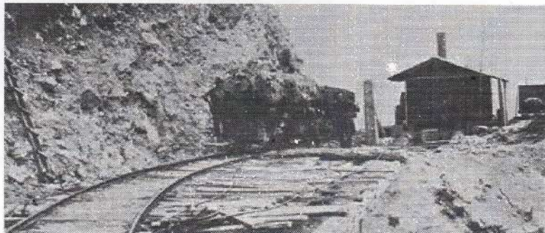
Figure 8: Hauler shed at top of Billygoat incline, housing a Judd steam winch that had extra braking to help control the descent. In addition, a brakeman rode on the rear of the wagon.
