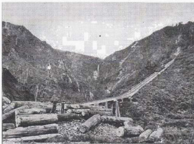
Figure 15: View of Billygoat Landing, with empty bogeys being winched up the incline. Billygoat Falls are near the centre and smoke from the steam winch boiler can be seen towards the top right.
