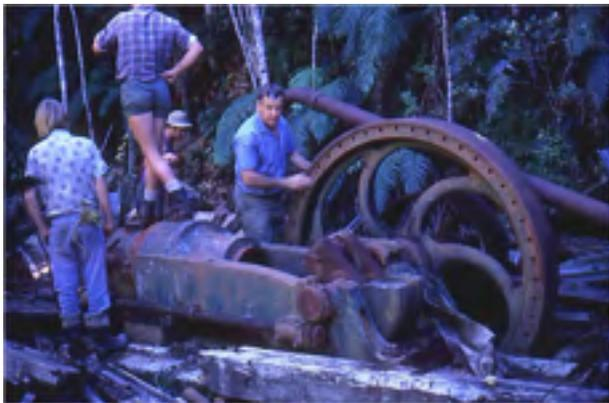
The Neavesville Battery is located and dug into what is effectively a cliff face. Above the Battery and further up the hill is a "chimney" with an adit at the bottom. This was a "dry" Battery with little water available for processing the ore. Wood was loaded into the "chimney" which was about 6 feet dia. and 30 feet deep and the raw ore was added on top of the wood. A good fire was then raised which dried the ore to a state when it could be crushed and processed. According to
