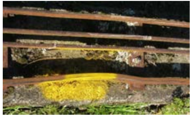
Damaged rail
